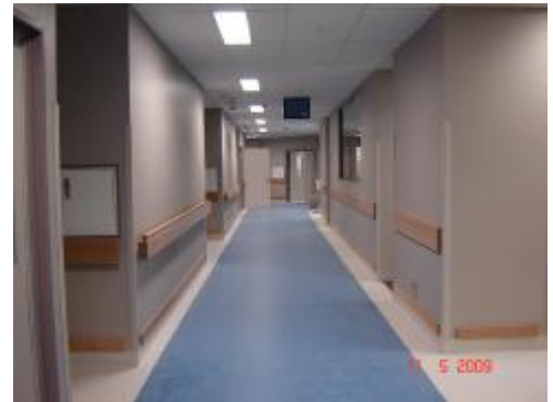
On completion Levels 2 and 5 will look similar to the ward above
