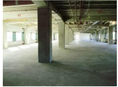
Level 2 is currently an empty shell.
