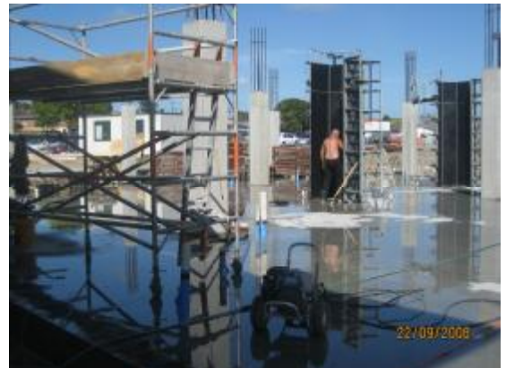
The floor slab has been poured for Building A.
