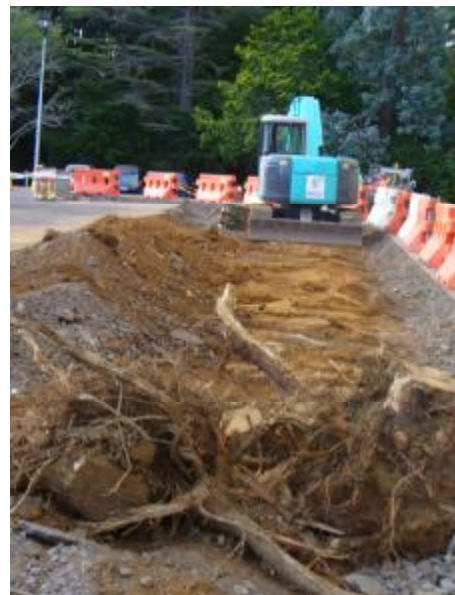
Kerbs and Islands are being worked on.
