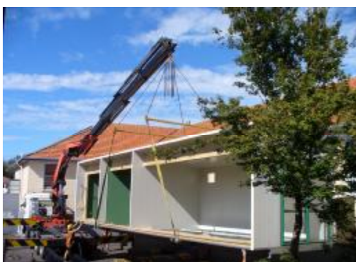
The Portacom weighing several tons is lifted into place
