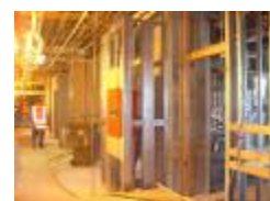
ANPN framing – west corridor
