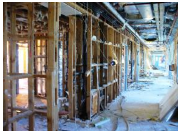
Ward 15 is being demolished in the Galbraith Building.
