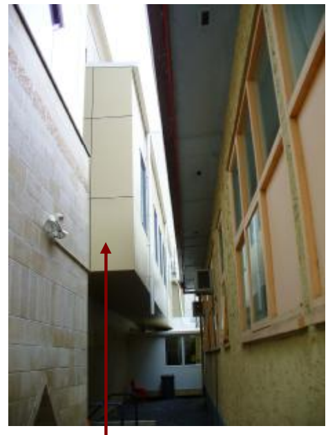
The corridor will link the future Intensive Care Unit (ICU), the existing C-Pod and National Burn Centre with the rest of the hospital.
