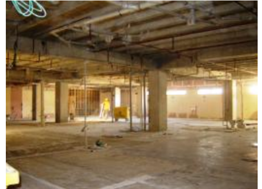
Demolition of old CCU
