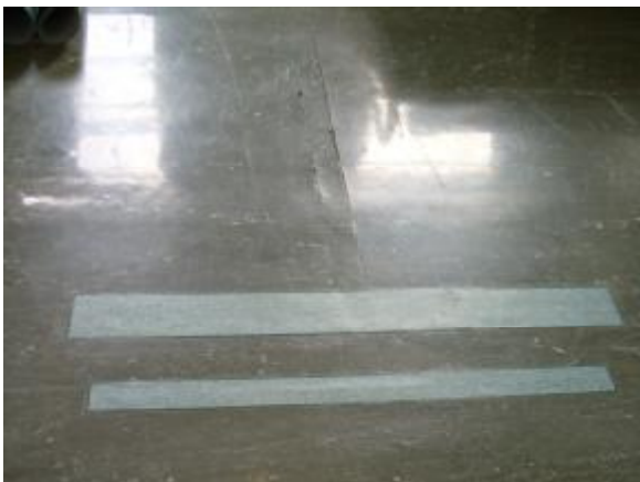
Cracked vinyl is being repaired
