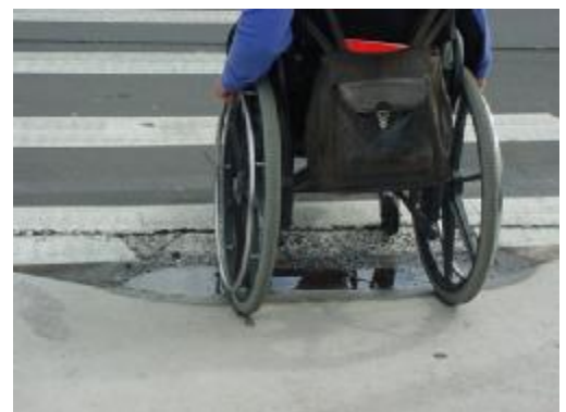
Kerbs will be fixed
