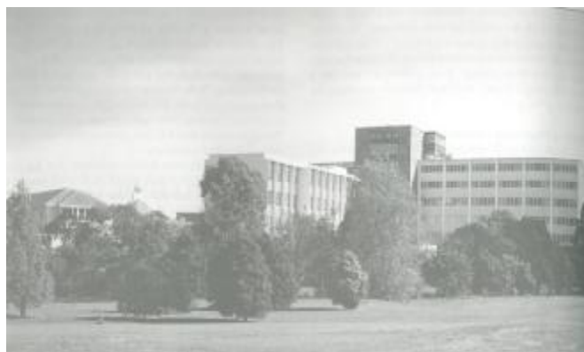
The completed Galbraith and Obstetric blocks from the Golf Course. These two buildings doubled the bed numbers of the Hospital.
