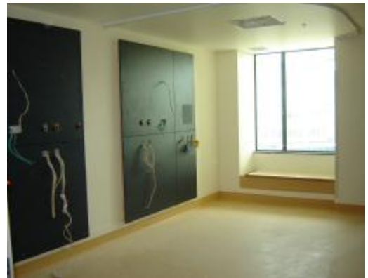
Construction photo of patient bedroom, 3 rd floor Medical ward.
