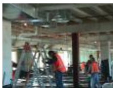
Builders install pipes and ducts, empty shell space - Level 3
