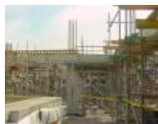
Construction of Level 4
