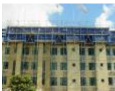
You can see the structural work for Levels 4 & 5
