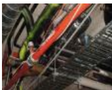
New pipes (red) replace old pipes (green and black)
