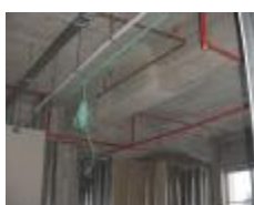
Installation of pipes and wiring
