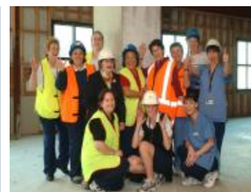
There's a buzz amongst the burn staff as they check out the first stage of construction of the National Burn Centre.
