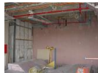
The installation of pipes, wires and ducts continue
