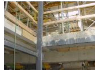
Looking up onto the 5th Floor
