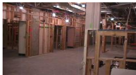
Demolition photo's – Stage 6
