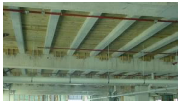
The AMC roof has been replaced with timber infills
