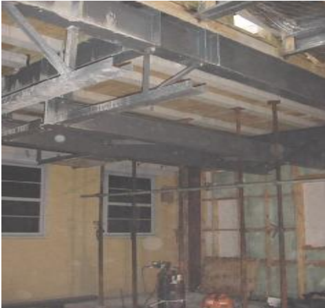
Steel beams suspended from the ceiling
