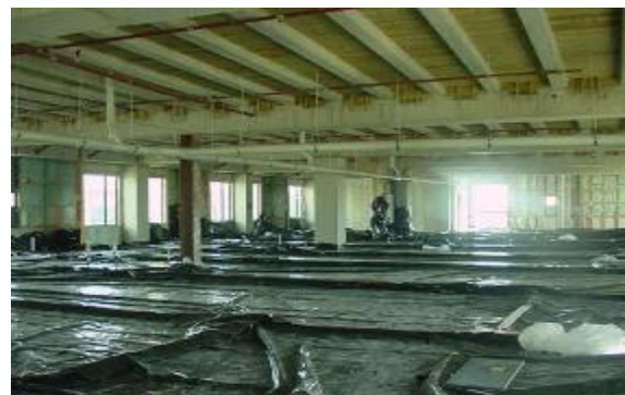
Waterproofing the floor – 'shell space' level 3, AMC.
