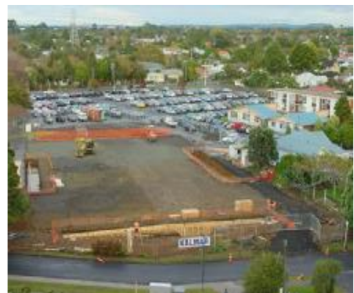
Groundwork preparation is complete July 2005
