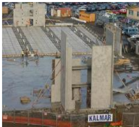
Structural framework in place August 2005
