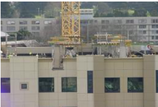
Workmen on the AMC roof
