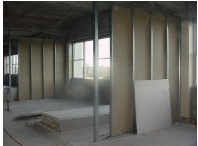
Plaster board being applied to the frames
