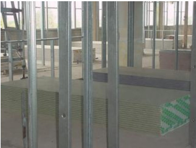
Steel frames for the walls
