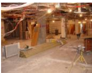
Stage R5 - Demolition Stage
