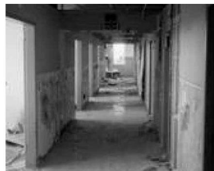
March 22nd – Walls Intact
